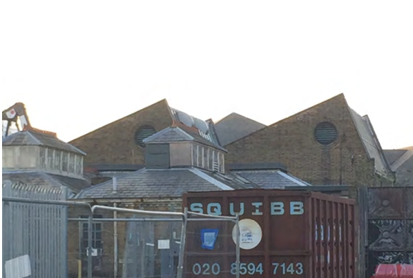
HISTORIC ROOF FORMS ON SITE
