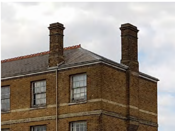
EXISTING ROOF FORMS ON SITE
