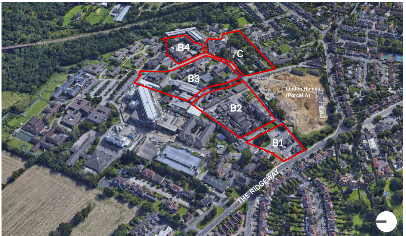
FIG 2 - AERIAL PHOTOGRAPHS FROM SOUTH AND WEST
