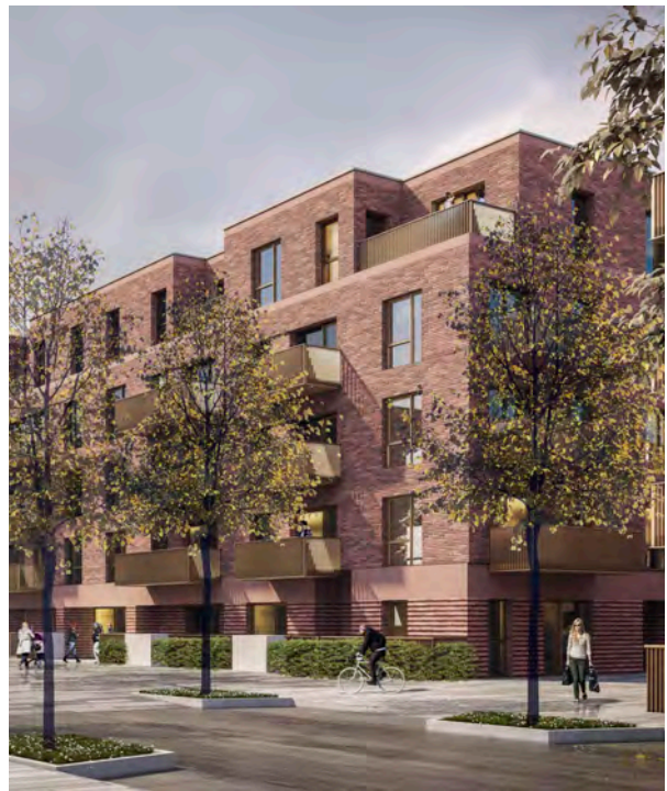
TERRACE BALCONY HARROW VIEW EAST - PTE
